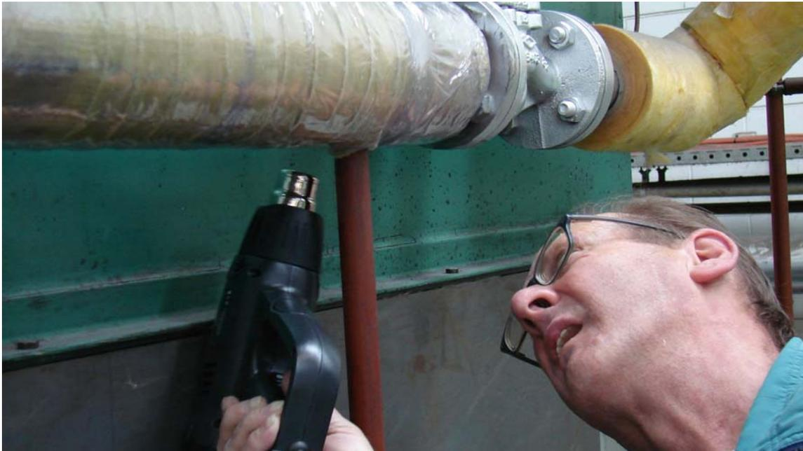
***Figure 5. Shrink wrapping the pre-prep to ensure air removal from the prepreg layers***
