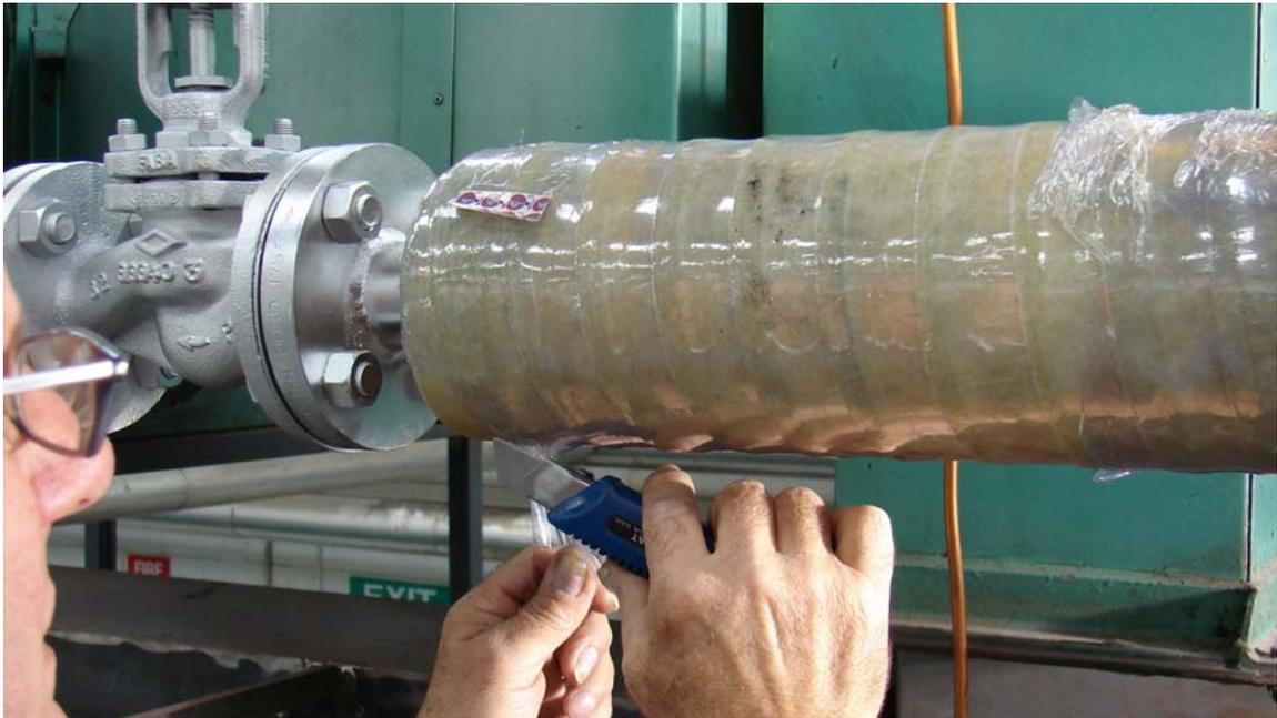
*Figure 6. Once cured, the plastic wrap is removed*
