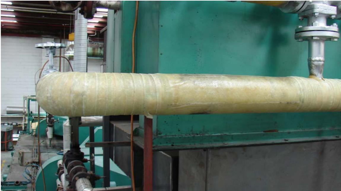
*Figure 7. – The completed UV curable pre-prep wrapped oil pipe*
