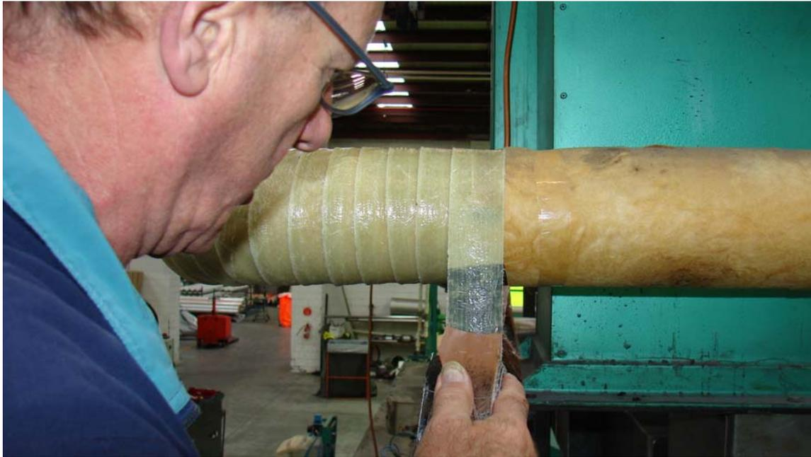
*Figure 3. – A technician applies the UV curable pre-preg in small over lapping strips over existing fibreglass.*
