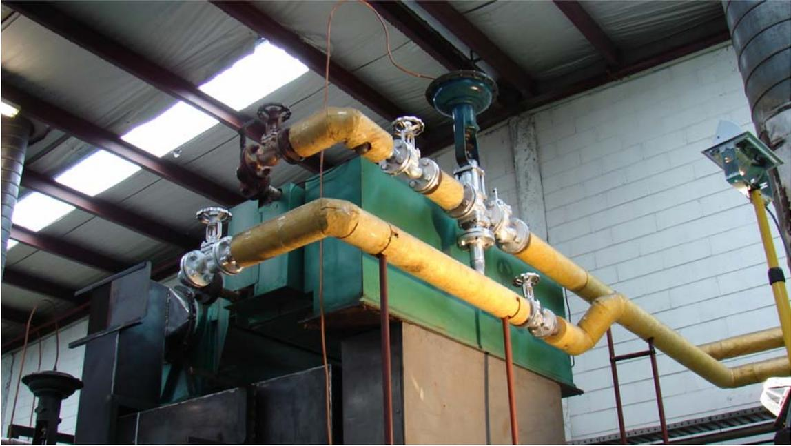
*Figure 1 – Wide shot of current insulation mounted over hot oil pipes*
