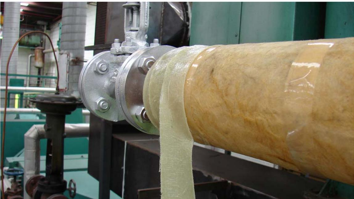
*Figure 2 – Auspreg UV #946 is applied in strips*
