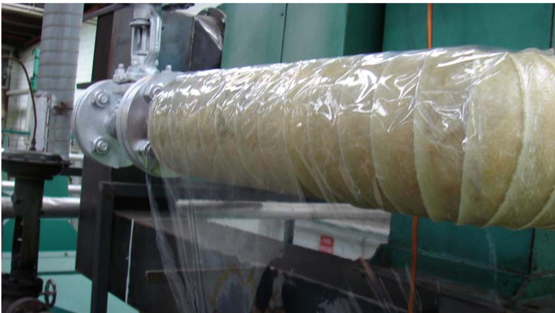
*Figure 4 – Shrink wrapping the pre-preg in anticipation for the vacuum process*
